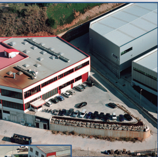
Arenys de Mar Plant
